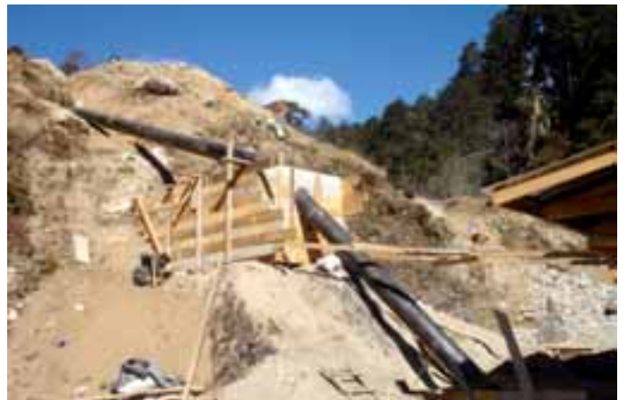
Construction of a penstock leading to the power house.
