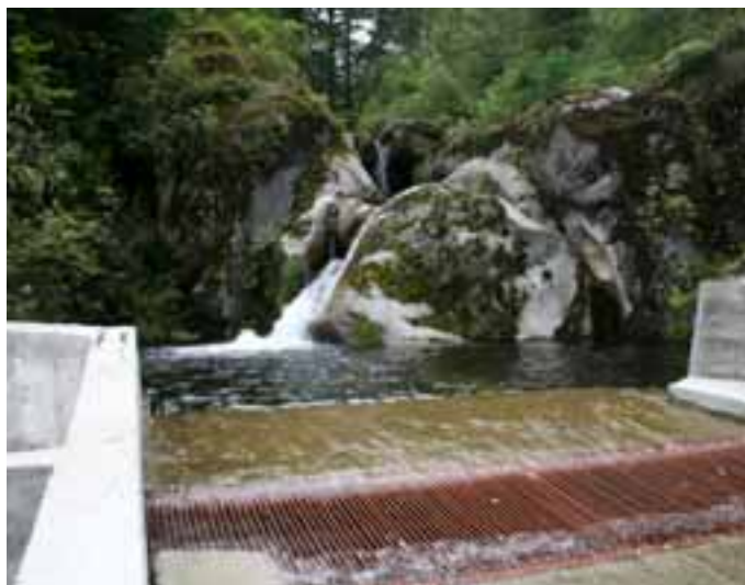
The intake reservoir after construction.
