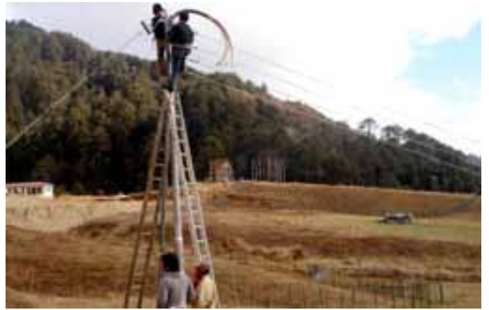
Construction of transmission lines.
