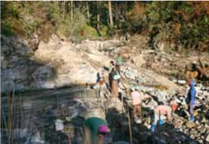
Construction of the intake reservoir.
